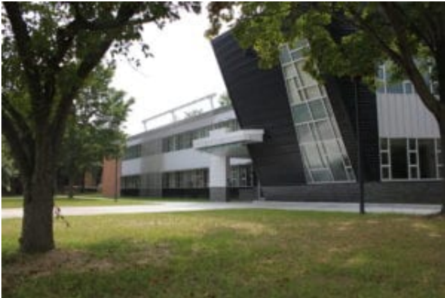
The Darwin R. Wales Center, one of the original campus buildings, underwent a dramatic renovation in Summer 2014.
