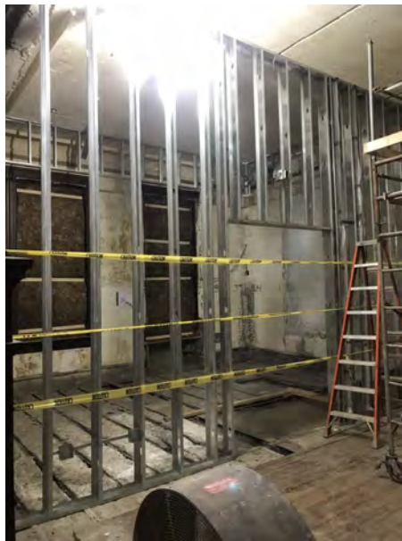
Progress on the future SUNY Broome Culinary Arts and Events Center: interior framing of the walls has begun in the historic Carnegie Library building!
