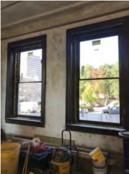
New windows at the Culinary & Events Center.
