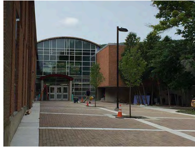
Work outside the Calice Advanced Manufacturing Center on Tuesday, Aug. 21.
