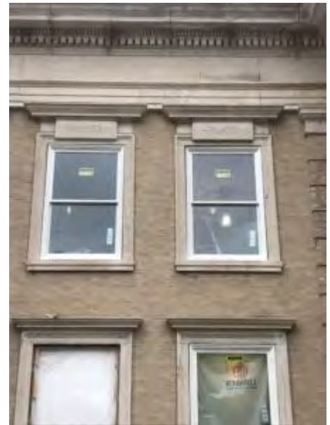
New windows at the Culinary & Events Center.
