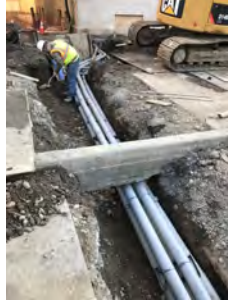
New electrical service installed at the Culinary & Events Center
