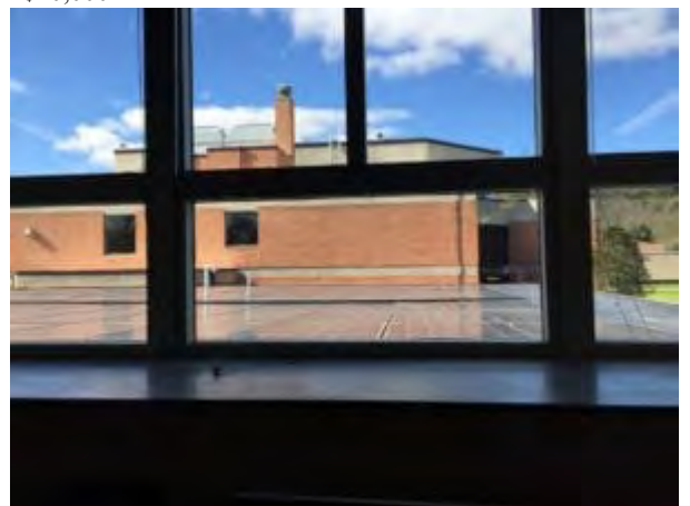
Solar panels on the roof of the Calice Advanced Manufacturing Center provide electricity.
