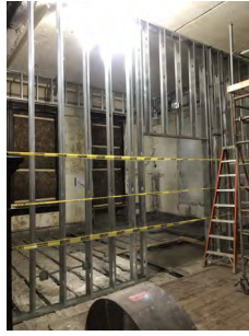
Progress on the future SUNY Broome Culinary Arts and Events Center: interior framing of the walls has begun in the historic Carnegie Library building!
