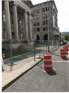
Work has begun at the former Carnegie Library site in Binghamton.
