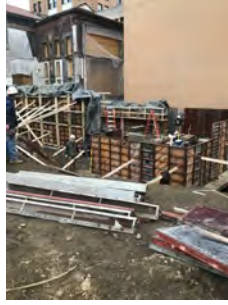
Walls being constructed for the new addition
