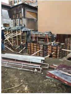
Walls being constructed for the new addition
