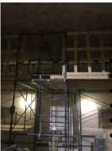
Plaster work in the grand staircase in the Culinary & Event Center
